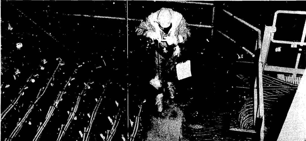
Figure 30. Technician performs radiation survey on control rod drive mechanism service structure platform.
