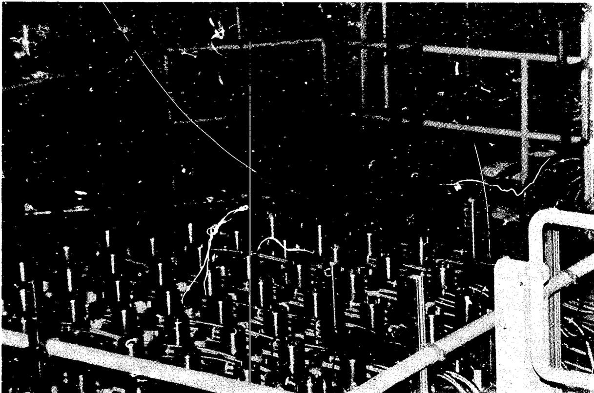
Figure 1. Relatively undamaged control rod drive mechanisms and associated cabling on the 347-ft elevation.
