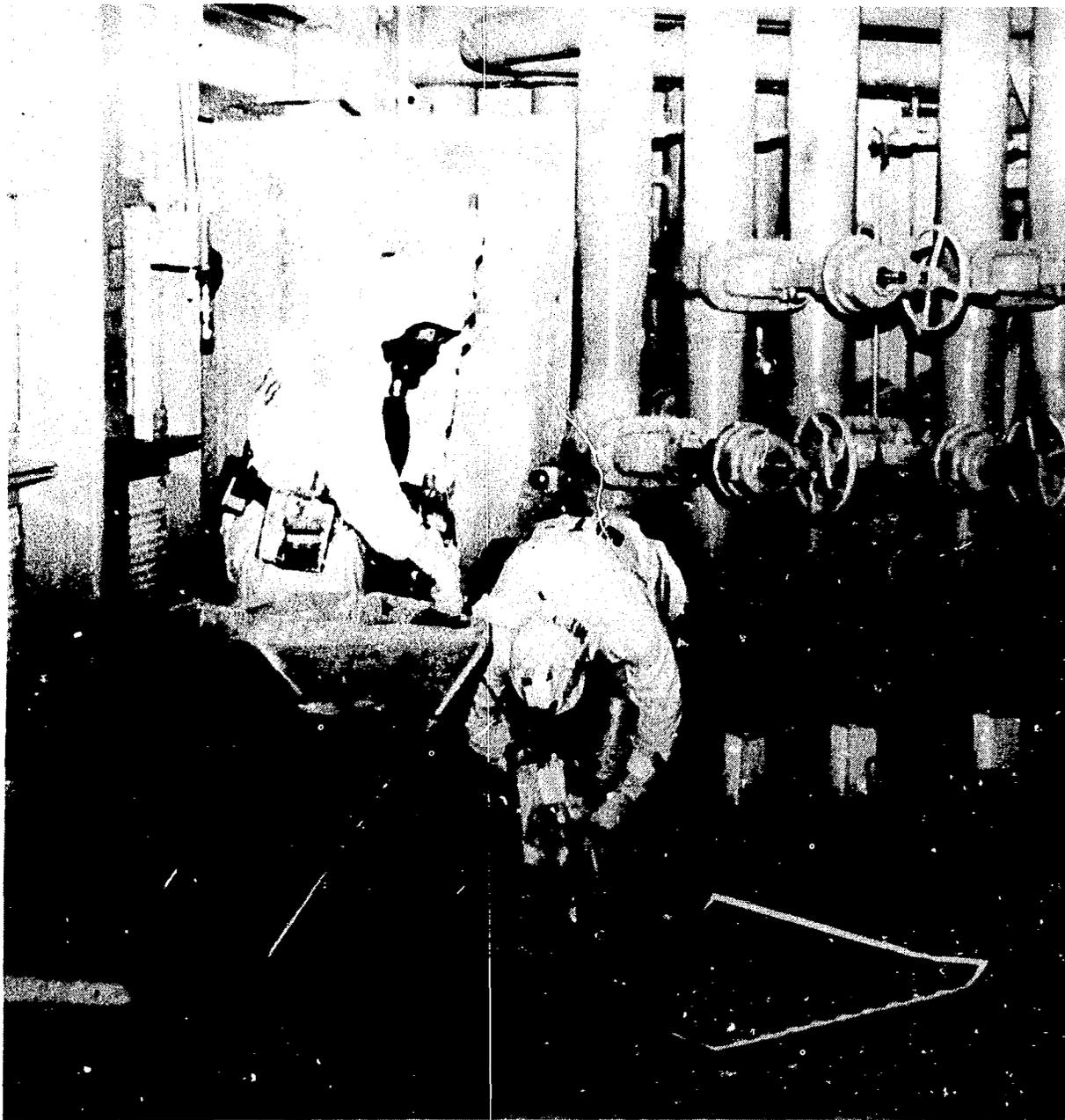
Figure 29. Technicians removing outer shoe covers at entrance to contamination-controlled area.
