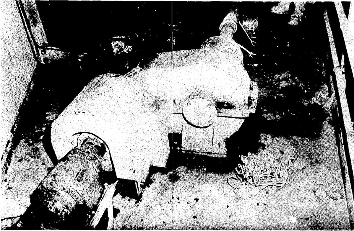
Figure 2. Corrosion and rust damage to polar crane motor and associated drive mechanism.
