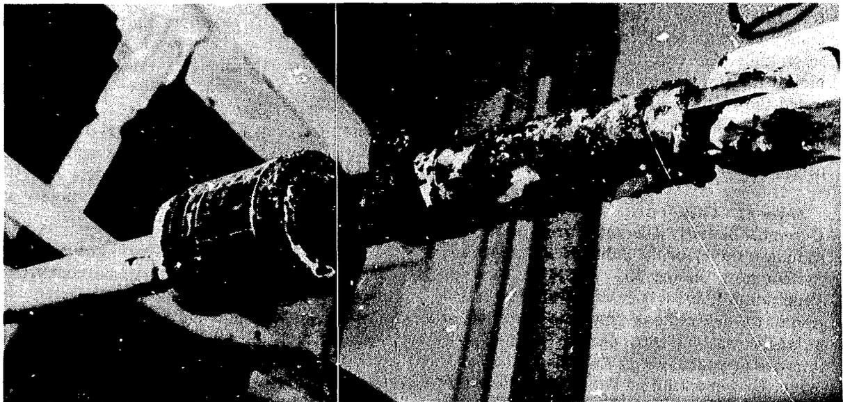
Figure 33. Corroded mechanical snubber on 305-ft elevation.
